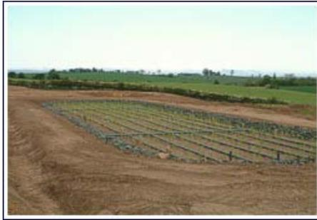
On the same site, alongside the reed-bed system, we have installed an ecologically friendly storm water run-off attenuation and treatment system comprised of, respectively, a Detention Pond and a Retention Pond to capture and treat all surface water run-off from the development site.
