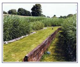
In the completed system the BioDisc was converted to a septic tank, settled effluent from this tank is pumped on demand to the 1st stage vertical flow reed-beds and two sludge drying reed-beds were installed to treat the sludge and solids that collect in the tank. Flowforms fitted to the first pond keep the water aerated and moving providing further treatment as well as an added attraction
