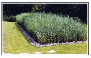
A new treatment system was required to replace an old BioDisc, increase the treatment capacity to cater for an expansion of the Leadership Trust's facilities at their Training Centre and ensure that the final effluent discharged to a stream did not exceed 23,000 litres/day while meeting consent limits of 10:20 mg/l for BOD and Suspended Solids. A robust, flexible system was clearly required to treat and balance flows that varied between 4,000 - 34,000
