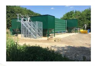
to ensure it worked to its fullest potential. In that time it became apparent that the original design figures under-estimated the loadings expected. A number of modifications, such as the addition of floating aerators, and another SAF Plant beside Pond 2, were made and some extra plant was added by others, especially to deal with the high ammonia levels.
